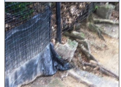
Damage in Small-Dog Run
